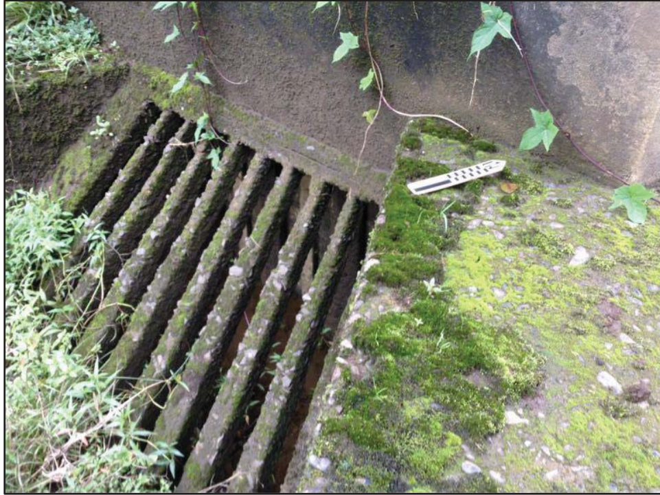
Figure 57. Close-up view of a concrete grate at the East Wailuanui Iki sluice gate, view to west
