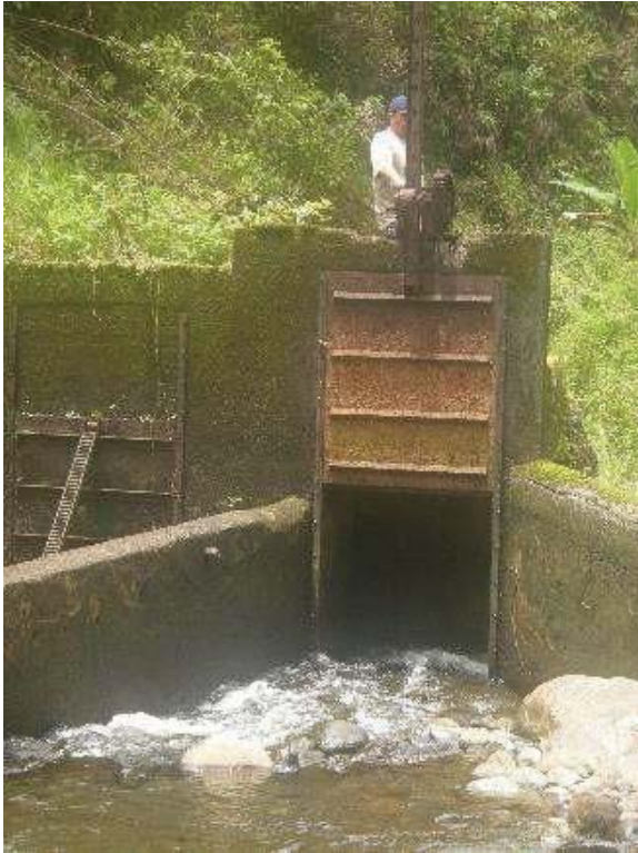
Figure 17: Geared sluice gate at Honomanu stream diversion dam. Eligible for the Hawaii Register as a contributing feature to a potential district. Integrity largely retained. View facing N. (Source: MAI, 2018)
