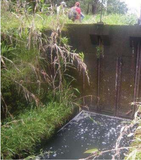
Figure 21: Threaded shaft sluice gate throw out (on left) at intake of Kolea Power House stream diversion. Eligible for the Hawaii Register as a contributing feature to a potential district. Integrity largely retained. View facing N. (Source: MAI, 2018)
