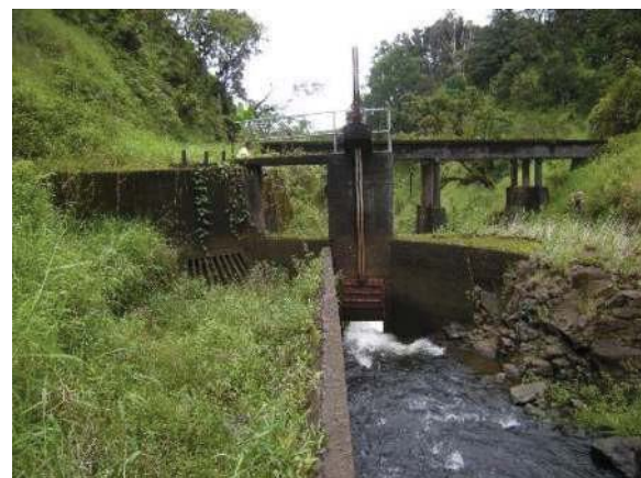
Figure 12: Ratchet sluice gate at Wailua Iki East stream diversion dam. Eligible for the Hawaii Register as a contributing feature to a potential district. Integrity largely retained. View facing NE. (Source: MAI, 2018)
