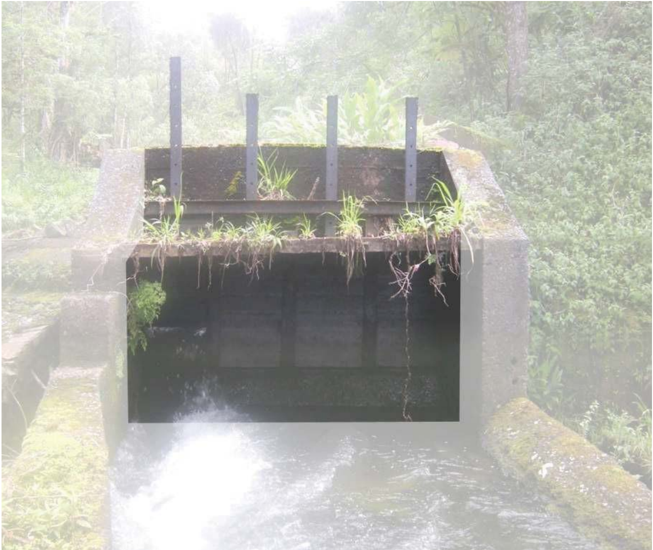
Figure 30: This typical board adjusted type sluice gate operating mechanism is located at EMI Kolea Power House stream diversion on Kolea, a tributary of Punalau, which is ordered to be restored as a “Habitat Stream” by CWRM. View facing SW. (Source: MAI, 2018.)
