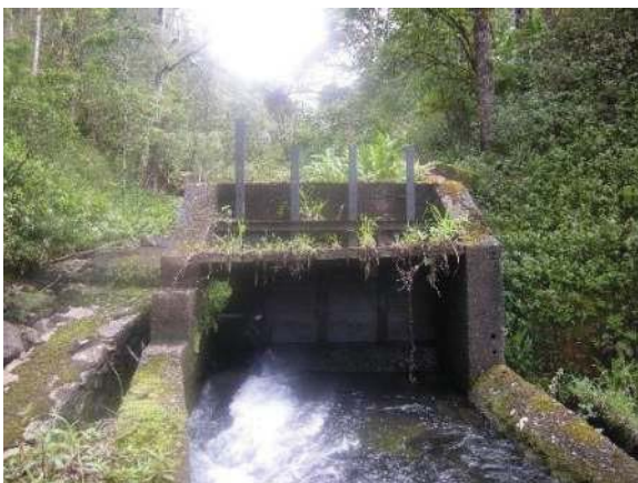
Figure 39: Board adjusted sluice gate at intake of Kolea Power House stream diversion. Eligible for the Hawaii Register as a contributing feature to a potential district. Integrity partially retained. View facing W. (Source: MAI, 2018)
