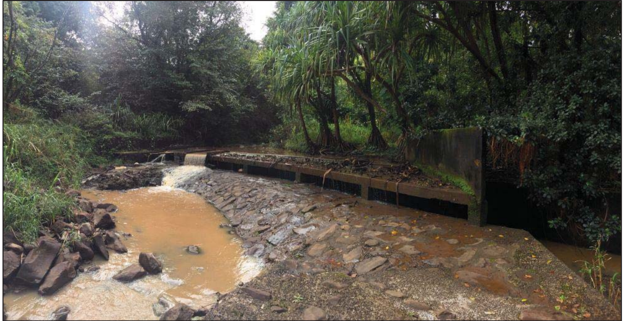
Figure 54. Honopou Stream diversion by Ha'ikū Ditch (CSH 2018)
