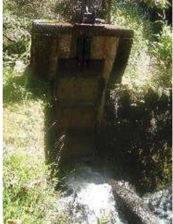
Figure 26: Ratchet sluice gate throw out at intake of Hoolawa Nui stream diversion. Eligible for the Hawaii Register as a contributing feature to a potential district. Integrity largely retained. View facing S. (Source: MAI, 2018)
