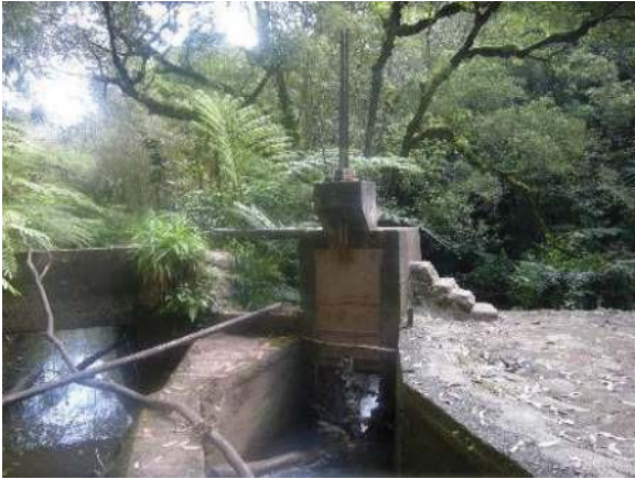
Figure 25: Ratchet sluice gate at Hoolawa Lii Lii stream diversion dam. Eligible for the Hawaii Register as a contributing feature to a potential district. Integrity largely retained. View facing NE. (Source: MAI, 2018)
