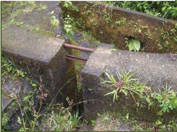
Board adjusted sluice gate throw-out at intake of Wai O Hue stream diversion. View facing SE.
