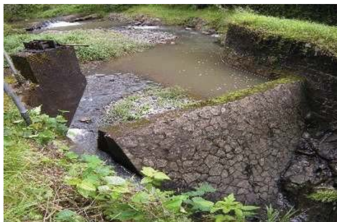
Figure 7: Dam at Wailuanui West Stream diversion impounds stream water for intake. (Source: MAI, 2018)
