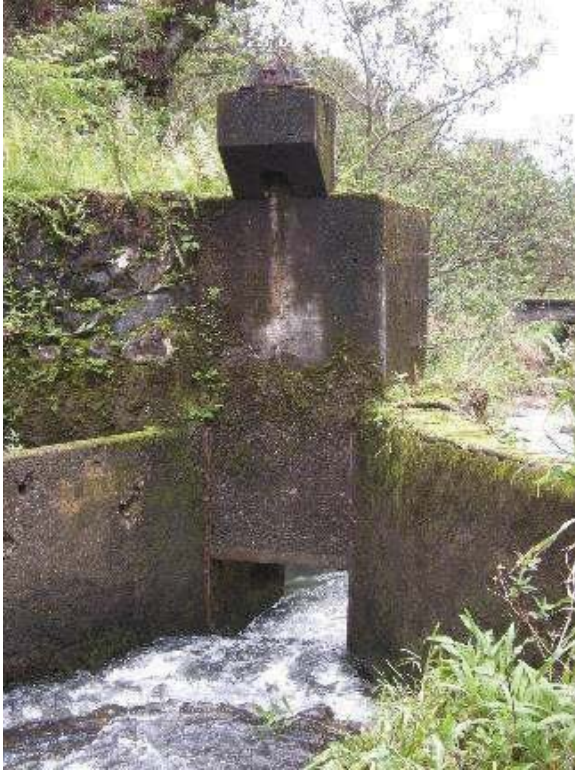
Figure 9: Removed sluice gate (ratchet) at Wailua Nui East stream diversion dam. Eligible for the Hawaii Register as a contributing feature to a potential district. Integrity largely retained. View facing NE. (Source: MAI, 2018)
