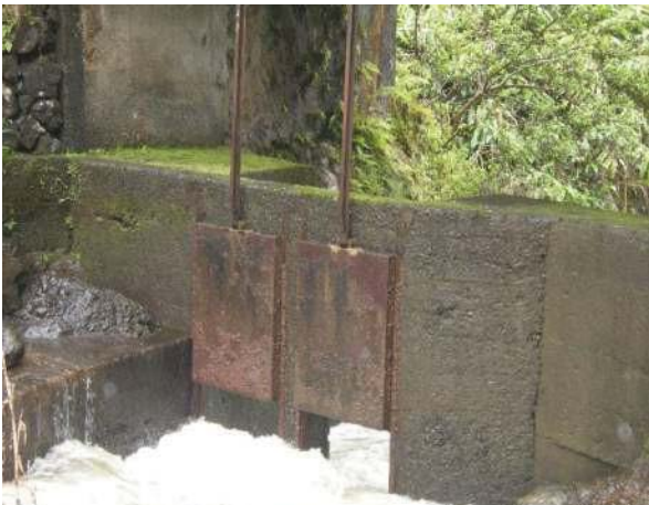
Figure 23: Typical board adjusted type sluice gate mechanism, shown with the gate closed. This gate is located at EMI stream diversion at Waiohue, which is ordered to be a “Fully Restored” stream by CWRM. View facing SE. (Source: MAI, 2018.)
