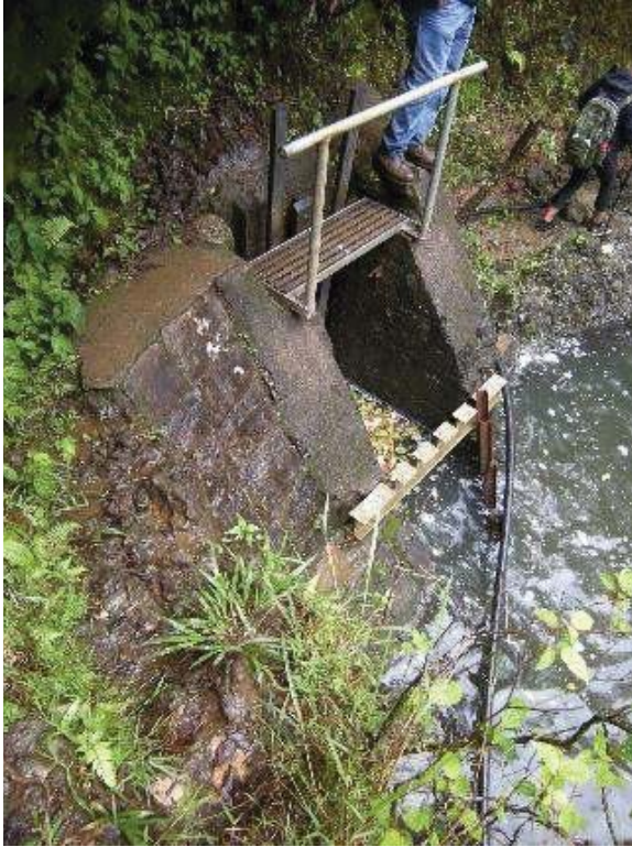
Figure 5: Board adjusted sluice gate at intake of Wai O Hue stream diversion. Eligible for the Hawaii Register as a contributing feature to a potential district. Integrity partially retained. View facing S. (Source: MAI, 2018)
