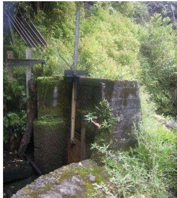
Figure 24: Ratchet sluice gate throw out at intake of Hoalua stream diversion. Eligible for the Hawaii Register as a contributing feature to a potential district. Integrity largely retained. View facing NE. (Source: MAI, 2018)
