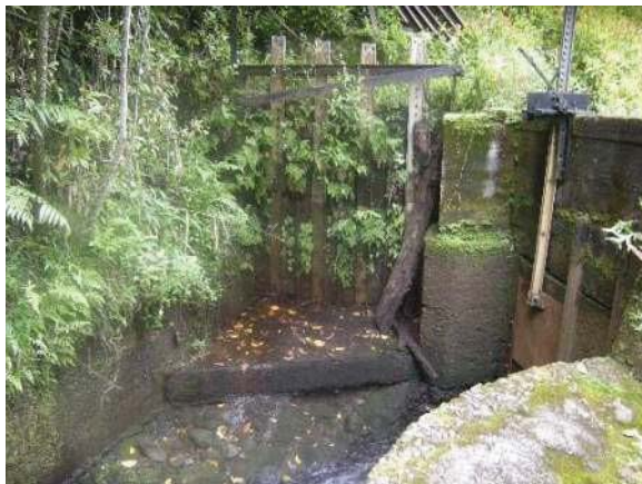
Figure 23: Board adjusted sluice gate (on left) at intake of Hoalua stream diversion. Eligible for the Hawaii Register as a contributing feature to a potential district. Integrity partially retained. View facing NE. (Source: MAI, 2018)
