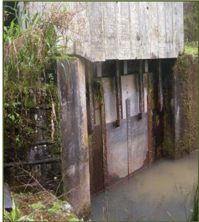
Geared sluice gate at intake at Ko Piliula stream diversion. View facing NE.
