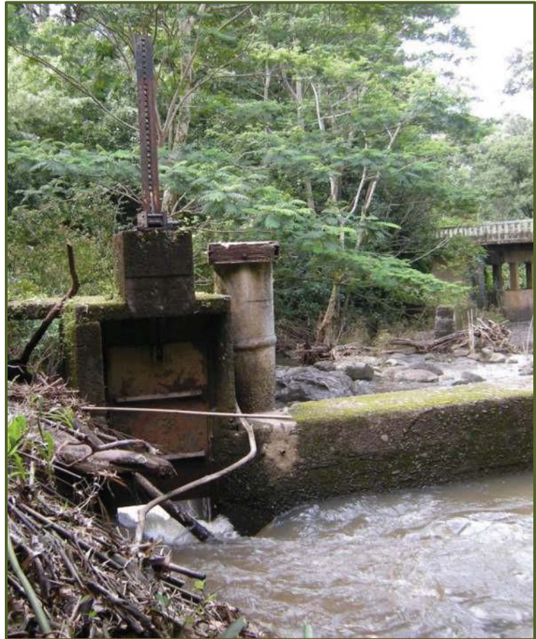
Ratchet sluice gate at Hanawi stream diversion dam. View facing SE.
