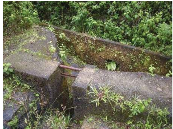
Figure 6: Board adjusted sluice gate throw out at intake of Wai O Hue stream diversion. Eligible for the Hawaii Register as a contributing feature to a potential district. Integrity largely retained. View facing SE. (Source: MAI, 2018)
