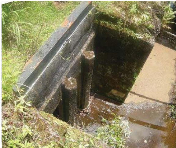
Figure 27: Board adjusted throw out sluice gate at Piinaau throw out. Eligible for the Hawaii Register as a contributing feature to a potential district. Integrity largely retained. View facing NE. (Source: MAI, 2018)
