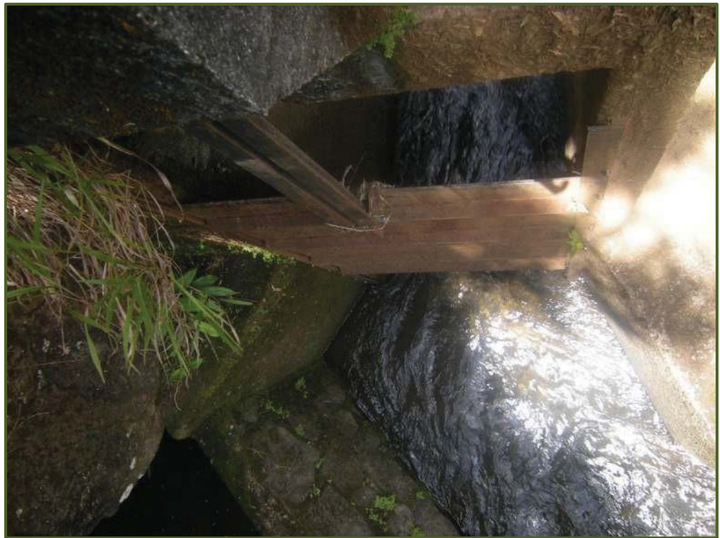
Ratchet sluice gate at Wai Ka Moi stream diversion dam. View facing NW.
