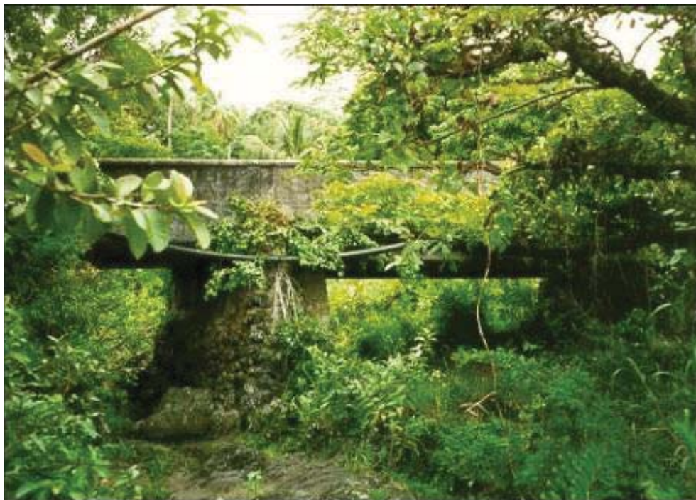
Figure 42. Papahawahawa Stream Bridge, a concrete beam and slab style bridge (Wilson Okamoto & Associates 2001)
