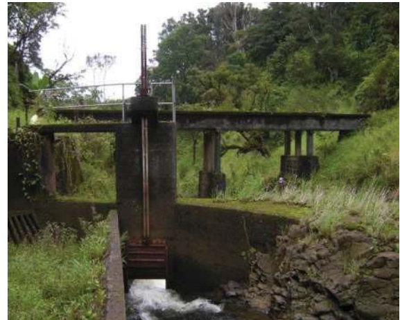
Figure 21: Typical sluice gate. Note the vertically sliding panel at the lower end that is operated by the mechanism above. This ratchet-operating gate is located at EMI stream diversion at Wailuaki East, which is ordered to be restored as a “Habitat Stream” by CWRM. (Source: MAI, 2018.)
