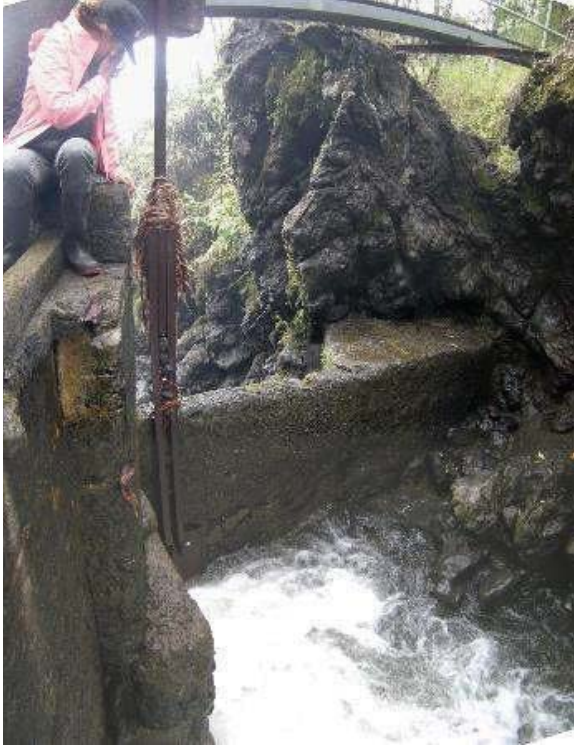
Figure 1: Ratchet sluice gate at Makapipi stream diversion dam. Eligible for the Hawaii Register as a contributing feature to a potential district. Integrity largely retained. View facing SE. (Source: MAI, 2018)
