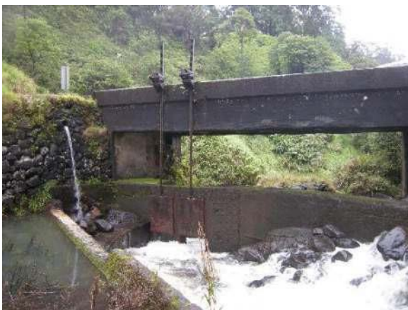
Figure 3: Geared sluice gate at Ko Piliula stream diversion dam. (Two sluice gates shown, side-by-side.) Eligible for the Hawaii Register as a contributing feature to a potential district. Integrity largely retained. View facing N. (Source: MAI, 2018)
