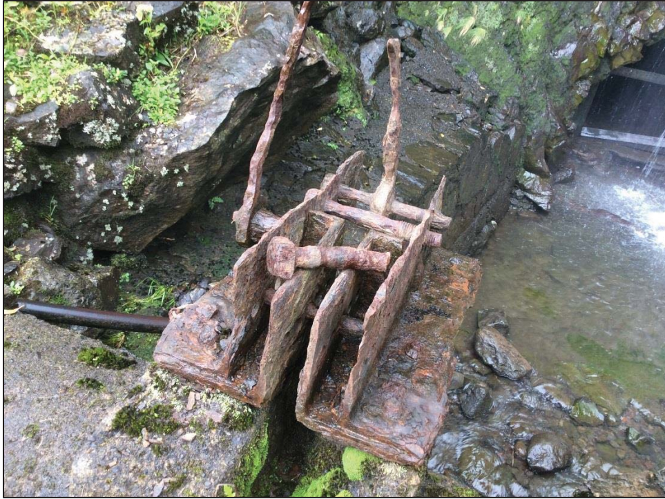
Figure 59. Close-up view of an abandoned iron sluice gate mechanism located along the ditch trail near the Banana sluice gate, view to southeast
