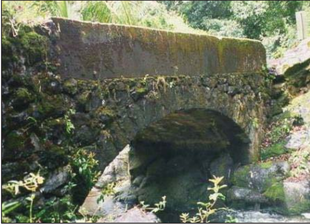
Figure 41. Hāhālawe Bridge, a characteristic masonry arch style bridge (Wilson Okamoto & Associates 2001)
