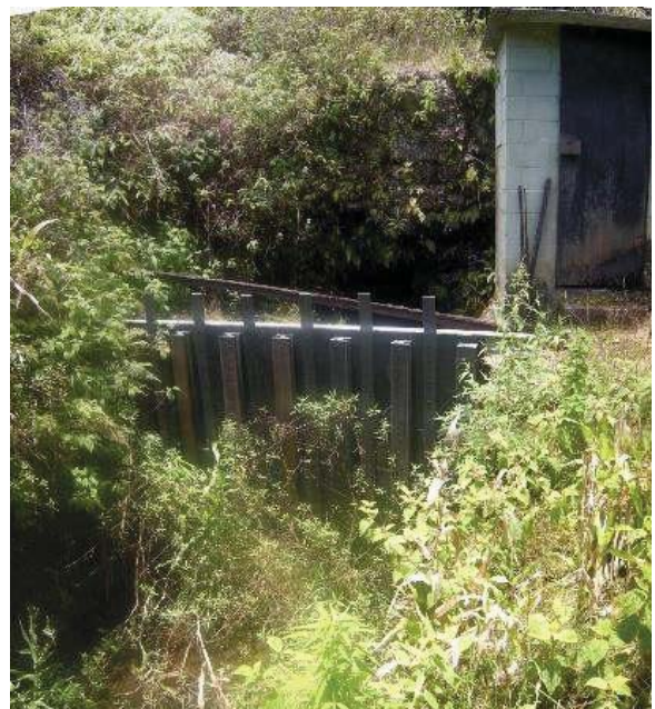
Figure 28: Board adjusted sluice gate at Piinaau throw out. Eligible for the Hawaii Register as a contributing feature to a potential district. Integrity partially retained. View facing SW. (Source: MAI, 2018)
