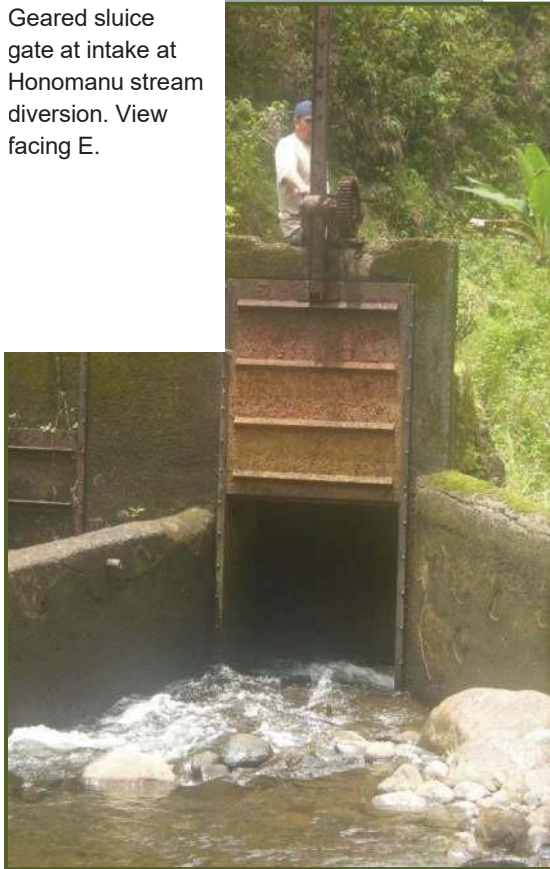
Geared sluice gate at Honomanu stream diversion dam. View facing N.
