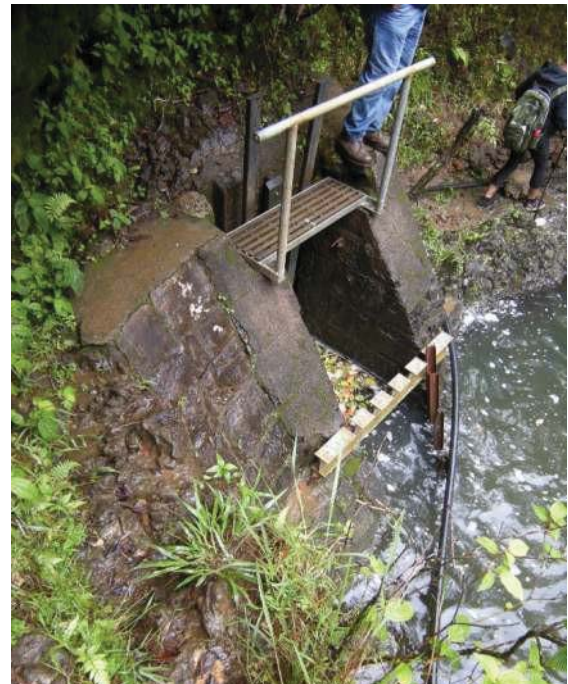
Figure 22: Typical configuration of sluice gates in a concrete dam. These sluice gates are located at EMI stream diversion at Kopiliula, which is ordered to be restored as a “Habitat Stream” by CWRM. View facing N. (Source: MAI, 2018.)
